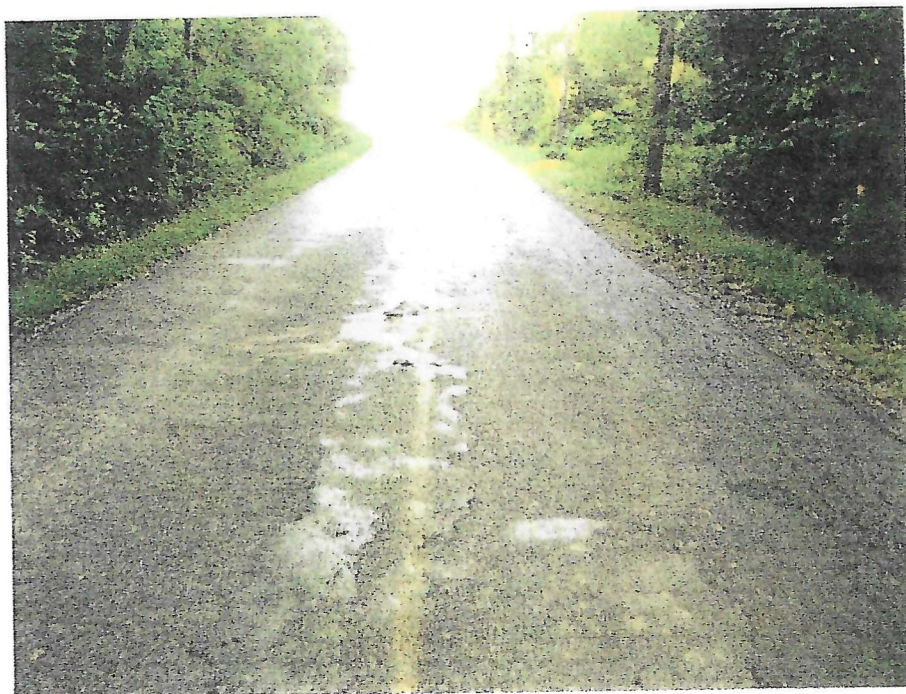
Raveling / Weathering – High Severity, Fatigue Cracking – High Severity
