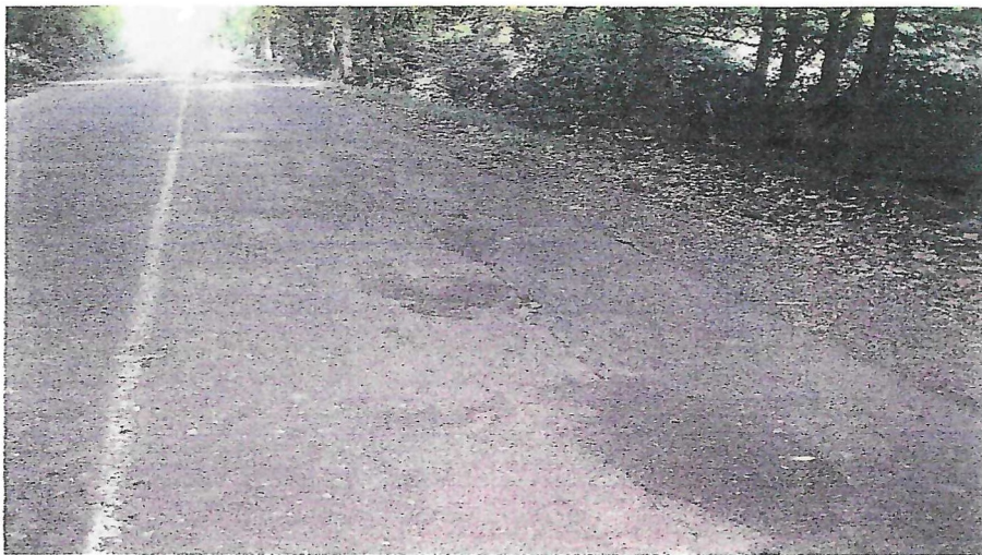
Fatigue Cracking – High Severity & Bituminous Patching
