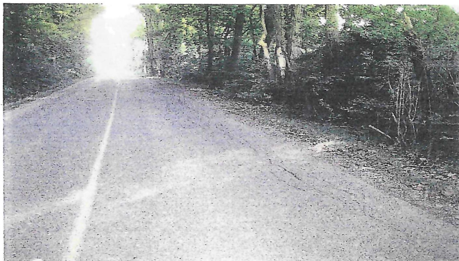
Fatigue Cracking — Medium Severity
