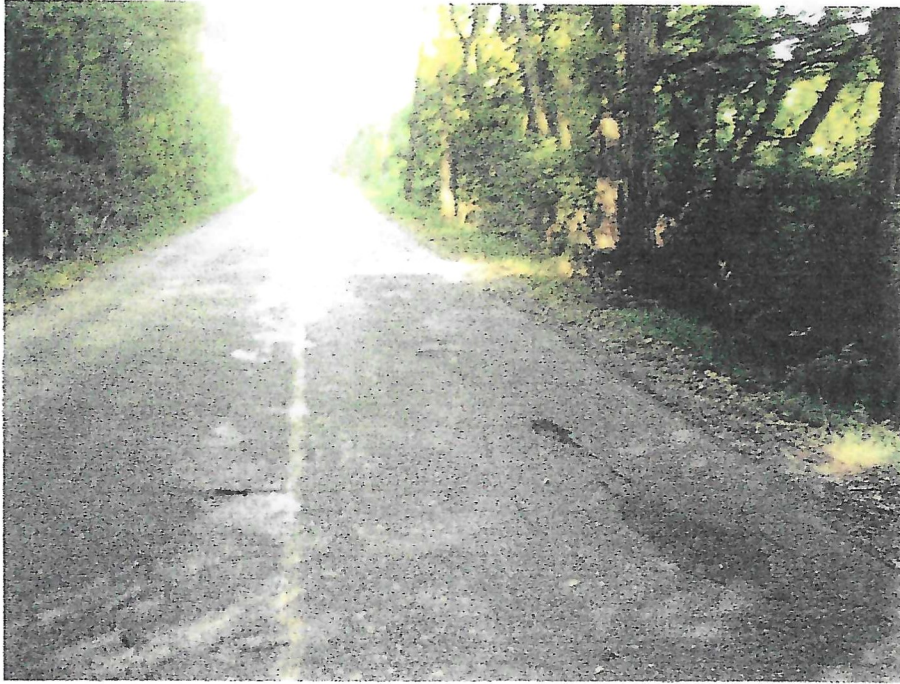
Raveling / Weathering – High Severity, Fatigue Cracking – Medium Severity & Bituminous Patching
