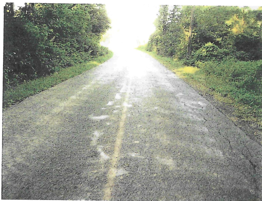
Raveling / Weathering – Medium Severity, Fatigue Cracking – Medium Severity
