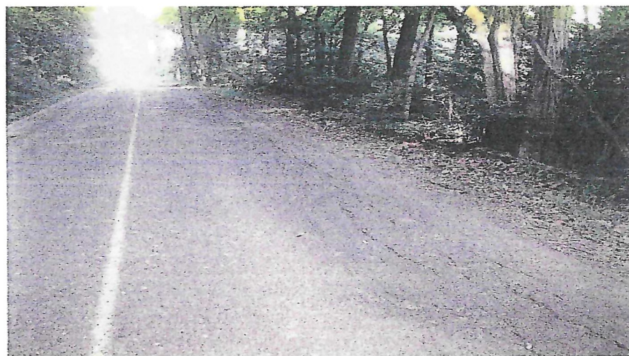
Fatigue Cracking — High Severity
