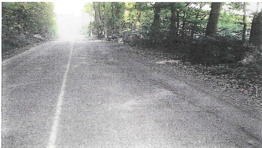
Fatigue Cracking – High Severity
