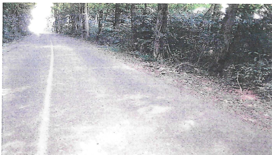
Edge Deterioration – Low Severity
