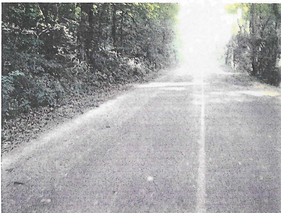
Fatigue Cracking – Low Severity & Raveling / Weathering – High Severity
