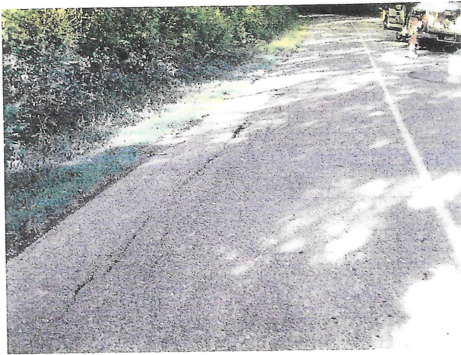
Fatigue Cracking – Medium Severity
