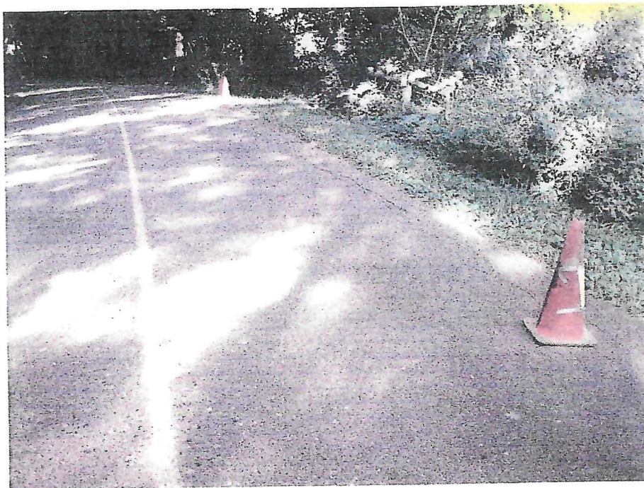
Edge Deterioration – Low Severtiy
