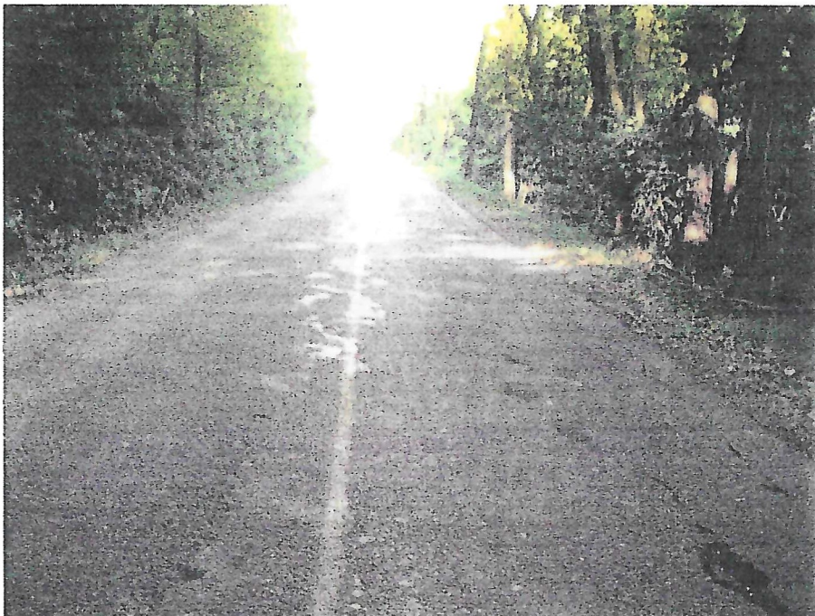
Raveling / Weathering – High Severity, Fatigue Cracking – Medium Severity & Bituminous Patching
