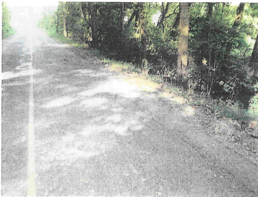
Edge Deterioration – Medium Severity
