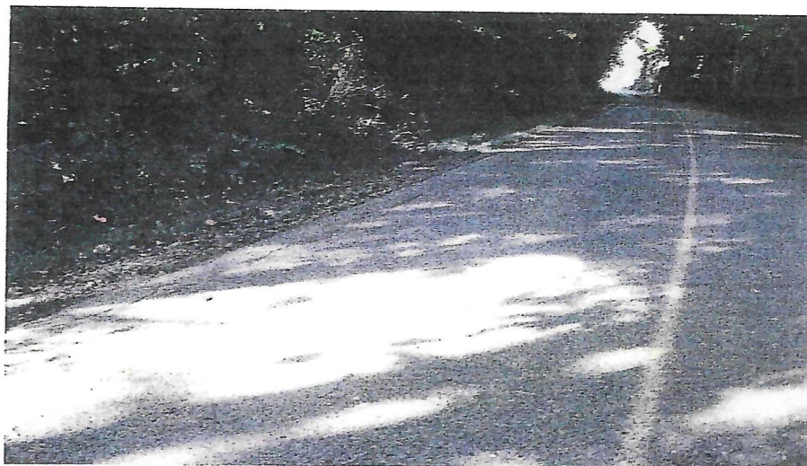
Edge Deterioration – Low-Severity
