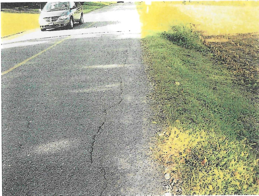
Fatigue Cracking – Medium Severity
